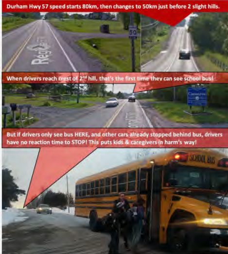
New Durham Highway 57 Common Stop where school bus stopping isn't visible until reaching crest of hill. Dangerous for Scugog Dead End Road Kids. Keep safer side road stops until turnaround can be built.
